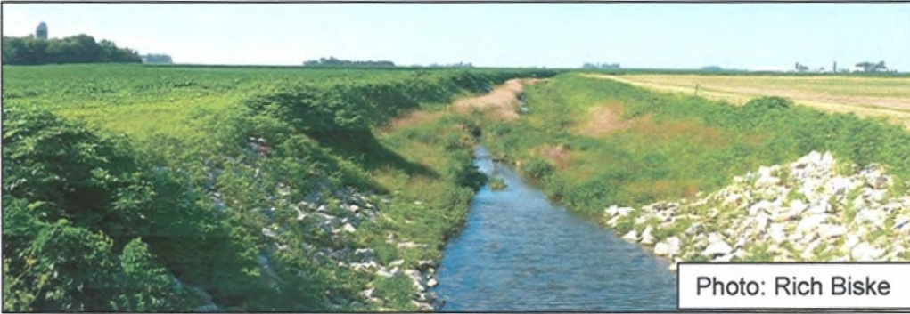
Figure 16. Upstream end 10 months following construction.
