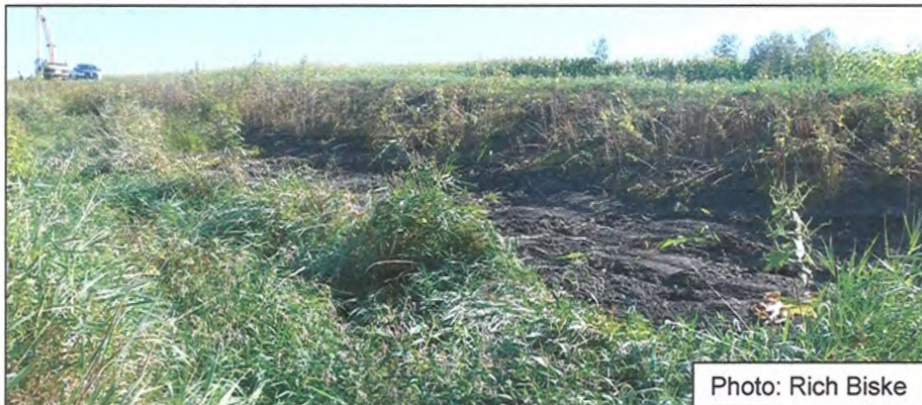
Figure 22. Repair of 2-stage ditch bank failure August 2010.
