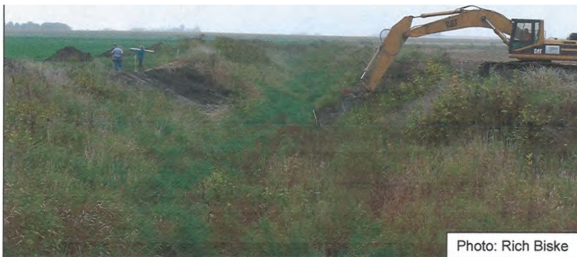
Figure 11. Upstream end during initial construction.
