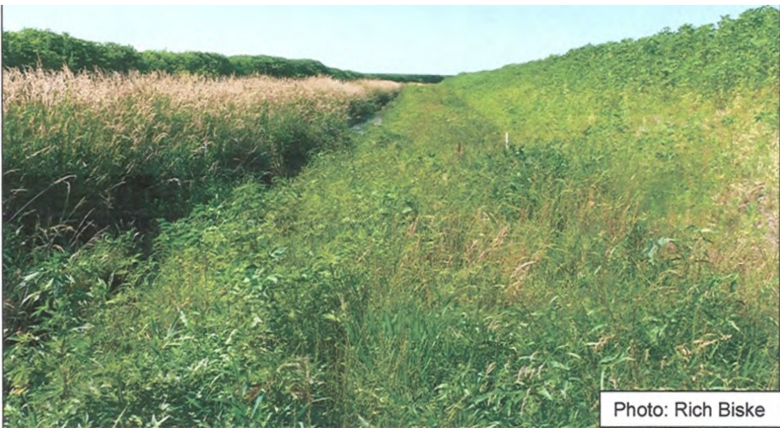
Figure 20. Stabilized 2-stage ditch bench June 2010.
