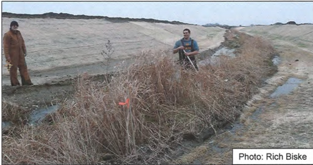
Figure 26. Installation of monitoring wells to measure seepage forces.
