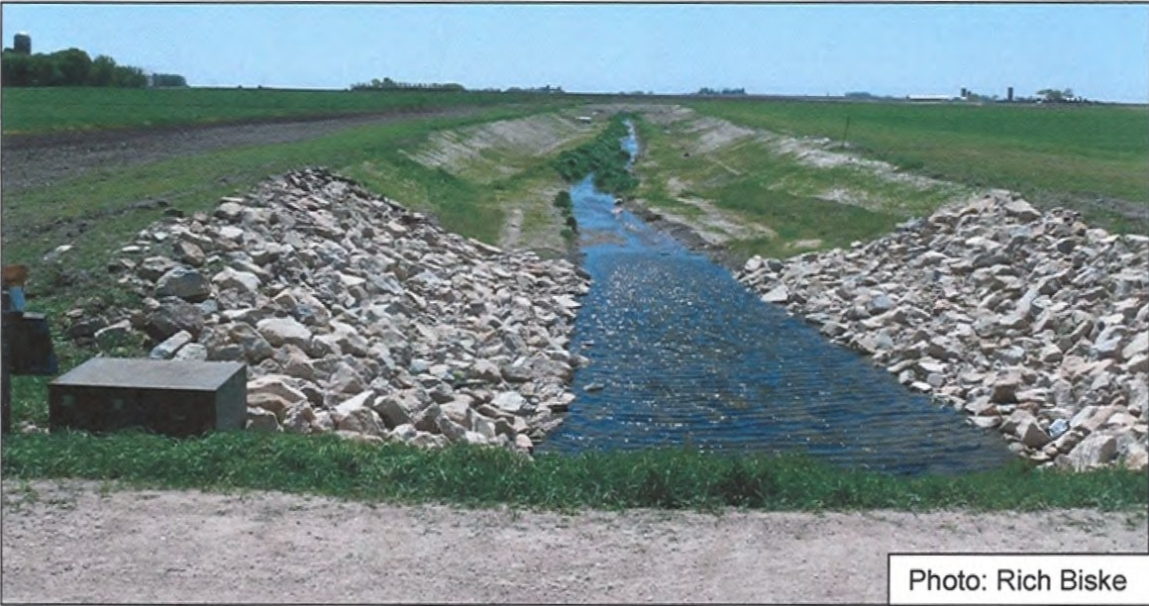
Figure 32. Monitoring station at upstream end of ditch.
