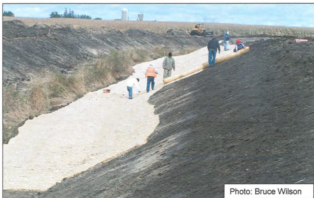
Figure 13. Placement of Erosion Control Blanket.
