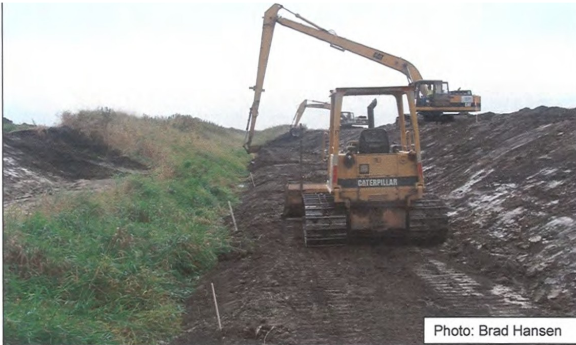
Figure 19. Stabilizing 2-stage ditch bench.
