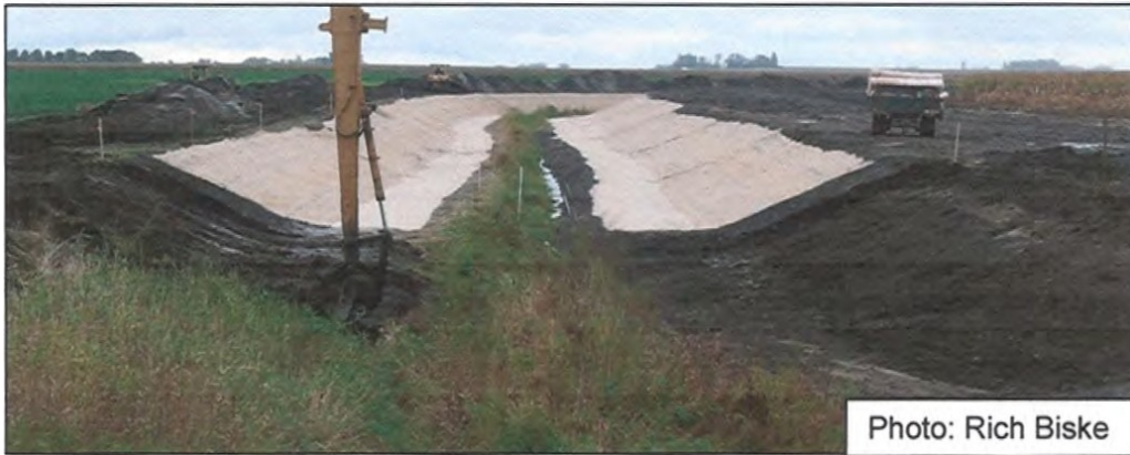
Figure 14. Upstream end during construction.
