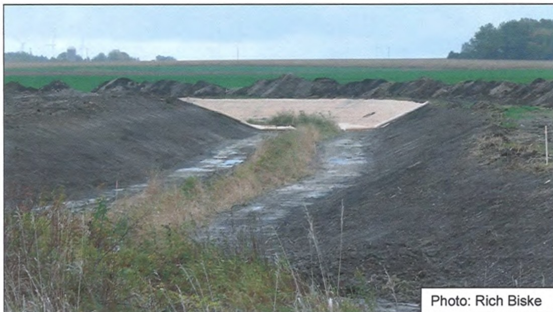
Figure 12. Excavated 2-Stage ditch showing vegetation in base flow channel
