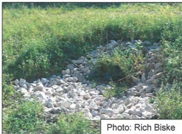
Figure 23. Rock inlet fixed with additional seeding and rip rap.
