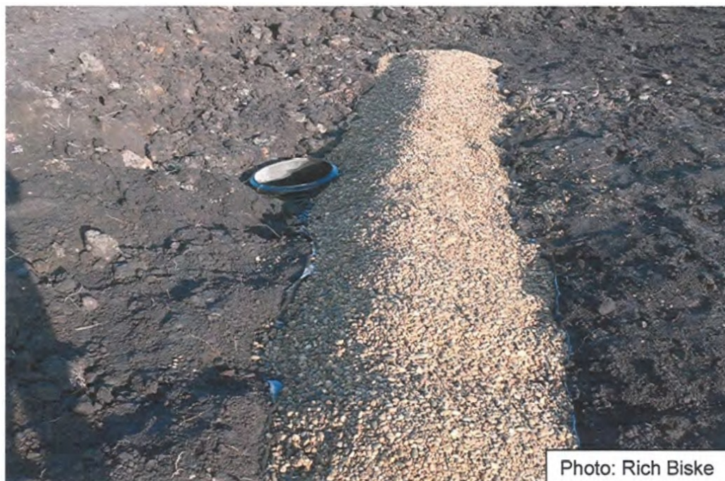
Figure 8. Top of modified side inlet showing rock lens.
