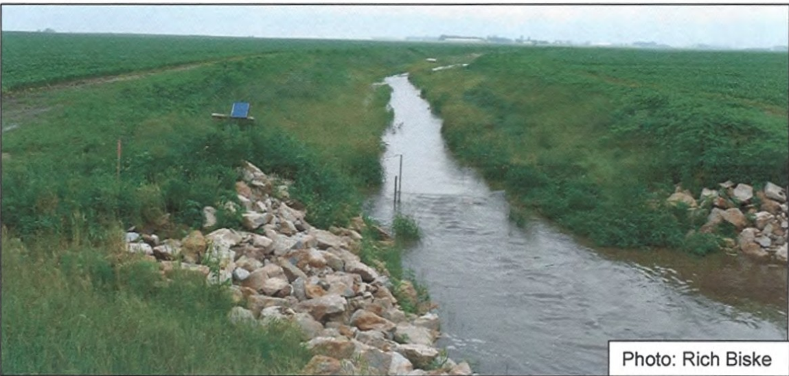
Figure 33. Monitoring station at downstream end.
